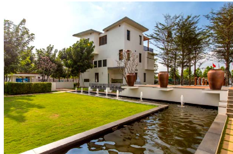
Completed villa at VNL's Dai Phuoc Lotus Island Project
