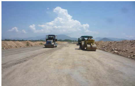
Resettlement Area – Road work
