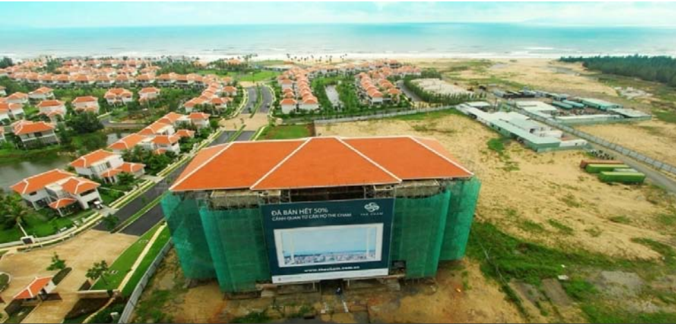
Current construction progress of the Ocean Apartment – Block A
