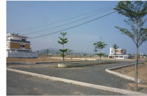
Phase 2.1 Internal works
